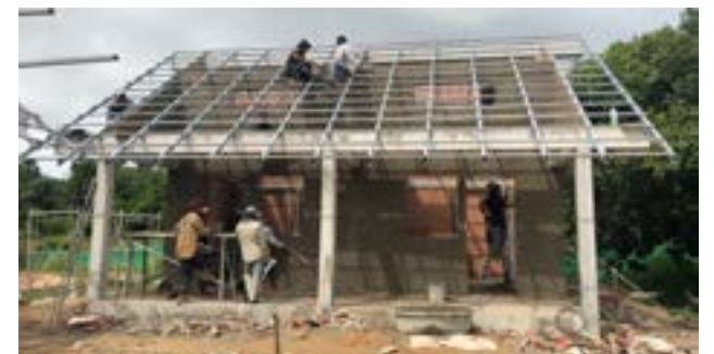
Construction begins on the SILA houses in Kep.
