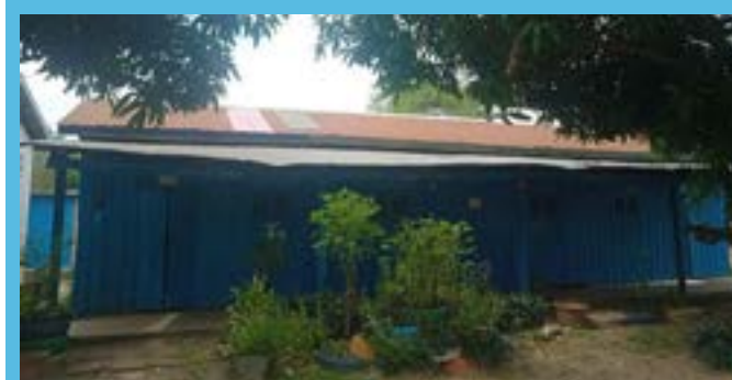
Original two-classroom NFE building 2003
