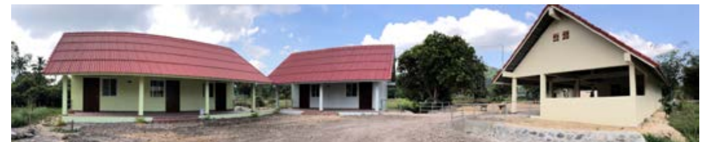
The three SILA houses after construction. In 2023, DT will transform the lawn into a lush common area.
